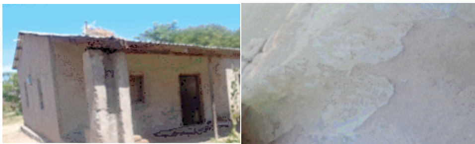
Figure 6: A beneficiary house in Chikwawa showing the effects of using low quality cement
