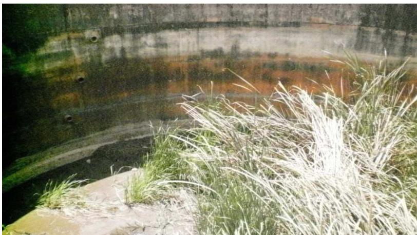
Picture 7: Blocked sludge digester at Zomba City Council waste water treatment plant (September 2011)
